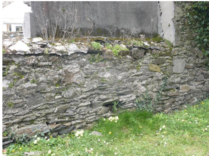
wall between Victoria Gardens and Malvern House
