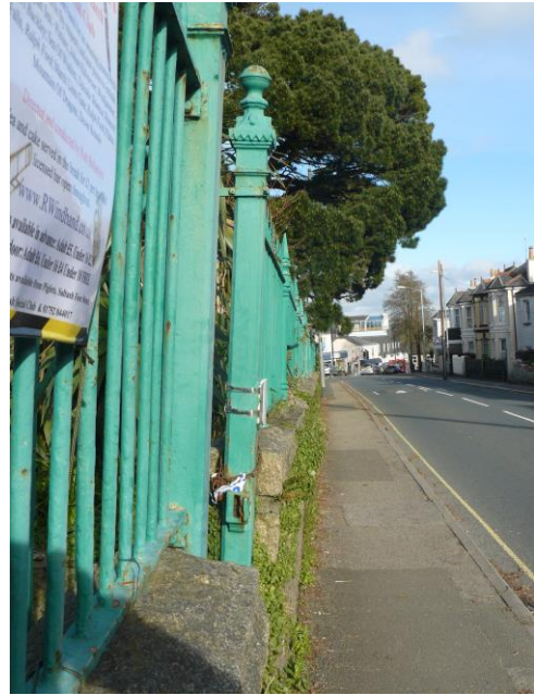
railing and wall leaning into St Stephen's Road
